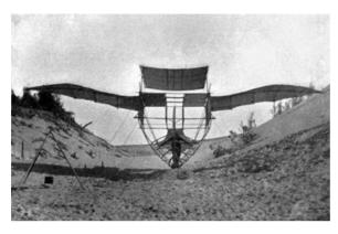
The *Albatross* was a large machine with a wing span of 40 feet and a wing chord of 7 feet. An 8 foot board ran along the bottom of the wooden fuselage. The pilot was supposed to be able to shift the center of gravity by running toward the front or back of the craft.
