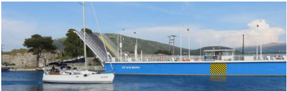
Floating bridge in Lefkada, Greece (images Dave Davey)
