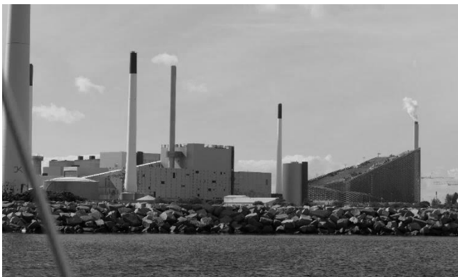
Copenhagen Fun-Fact: This powerplant burns garbage for fuel and part of its roof serves as a ski slope for this very flat country!
