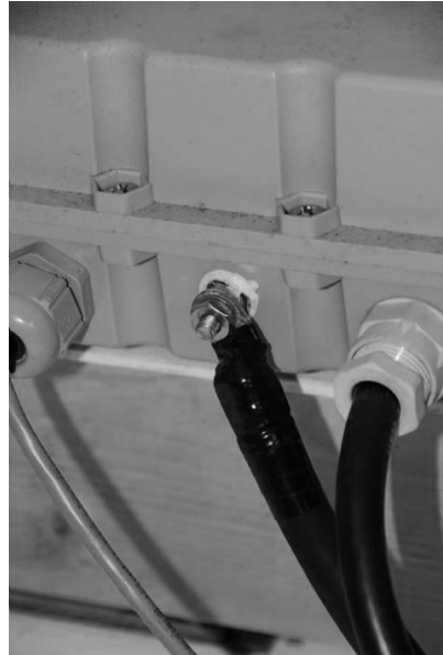
Figure 3: Radio frequency energy travels on the surface of cables, which is why copper foil is often used instead of wires. The effectiveness of the stud and standard cable would be reduced compared to a foil connection.
